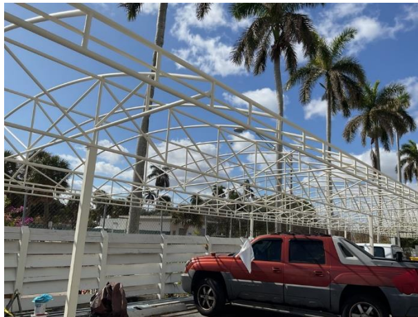
Awning with canvas being installed
