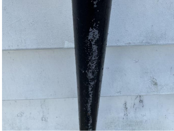
Finish deterioration
