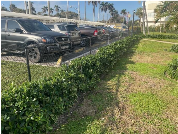
Chain link pool fence
