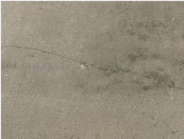
Wall cracks
