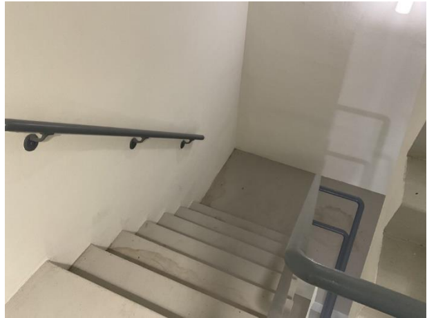
Stairwell paint finishes
