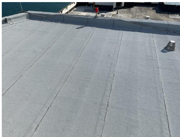
Modified bitumen roof overview
