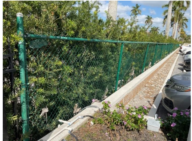
West perimeter chain link fence
