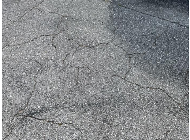
Pavement cracks
