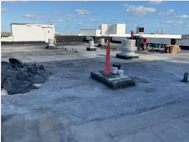
Coal tar roof overview
