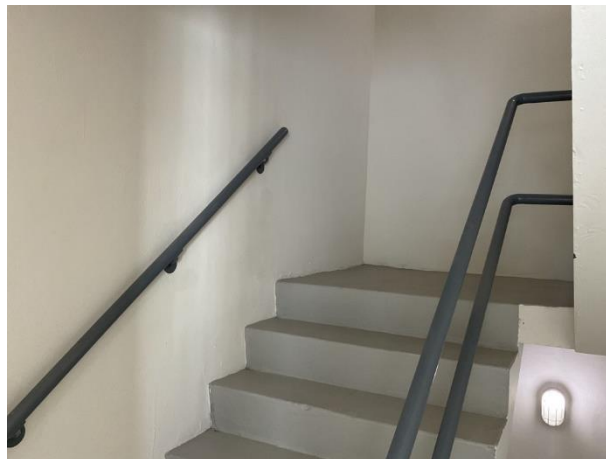
Stairwell paint finishes
