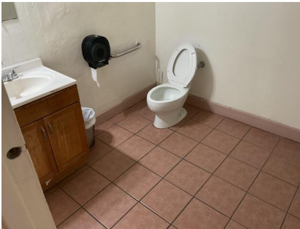
Main building rest room overview
