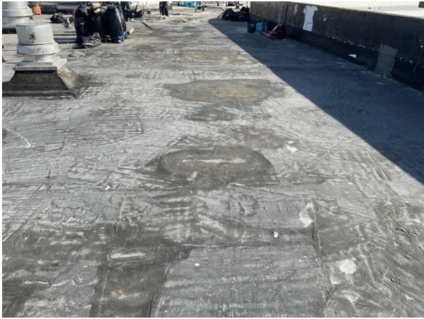
Coal tar roof overview
