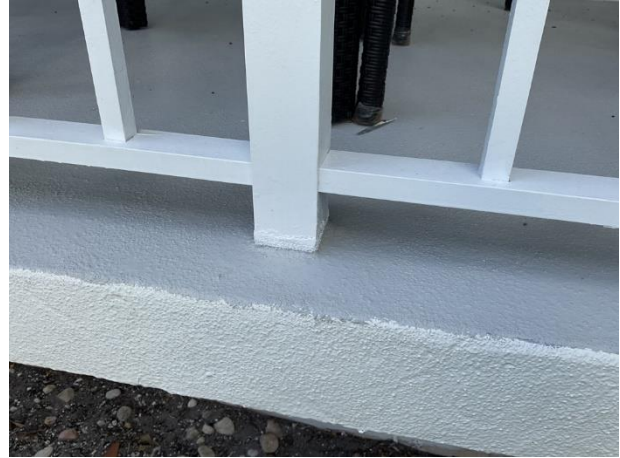
Railing post embedded in concrete
