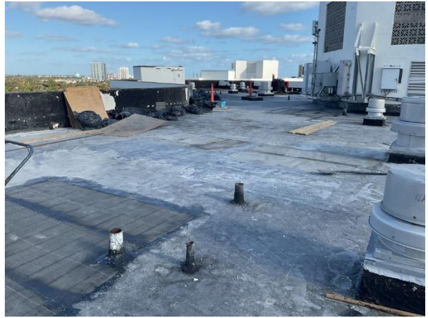
Coal tar roof overview
