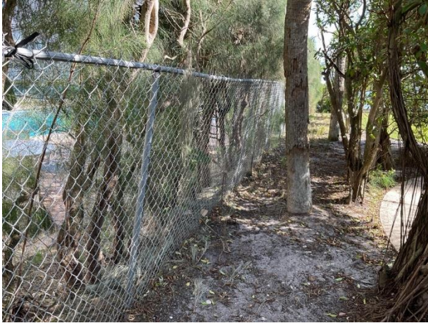
North perimeter chain link fence
