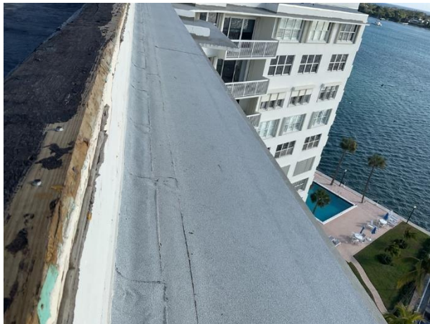
Modified bitumen roof overview
