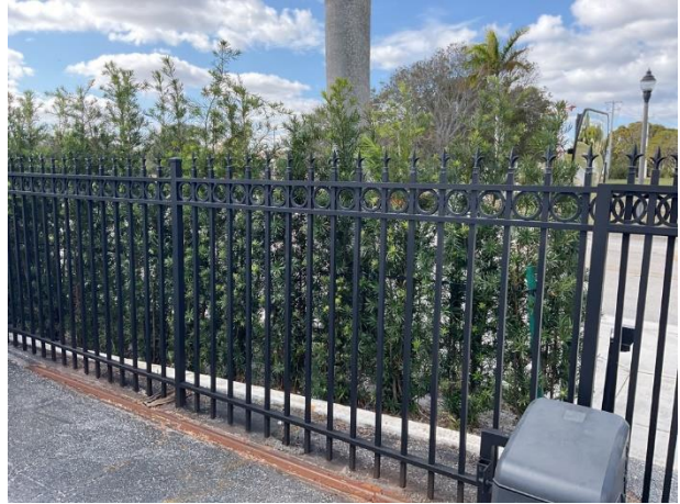
Fencing at gate
