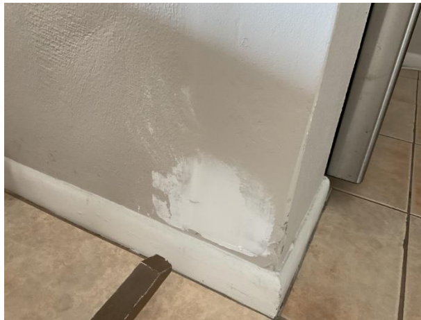
Previous wall repairs
