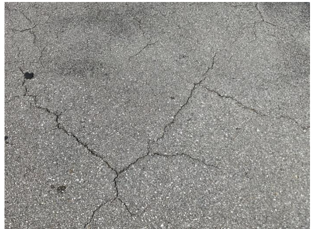
Pavement cracks
