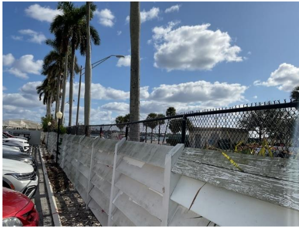
Chain link fence
