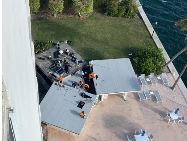
Modified bitumen roof at the pool house
