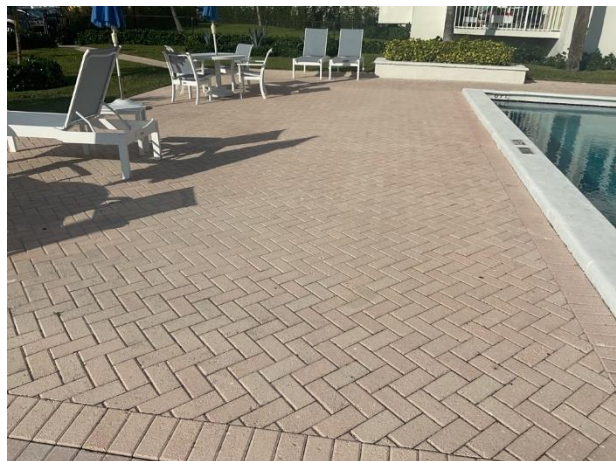
Paver pool deck overview
