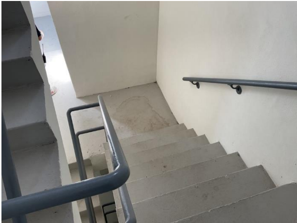
Stairwell paint finishes
