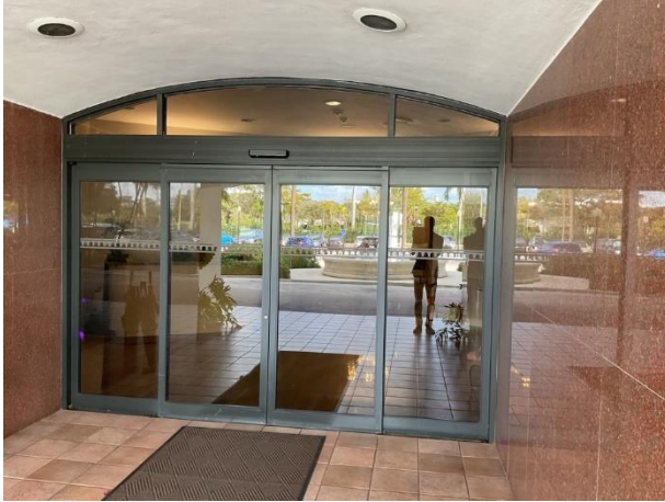
Lobby doors and windows
