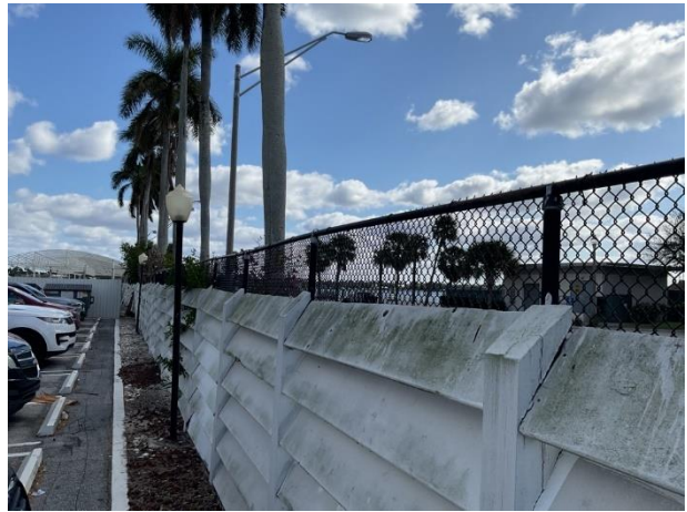
Chain link fence
