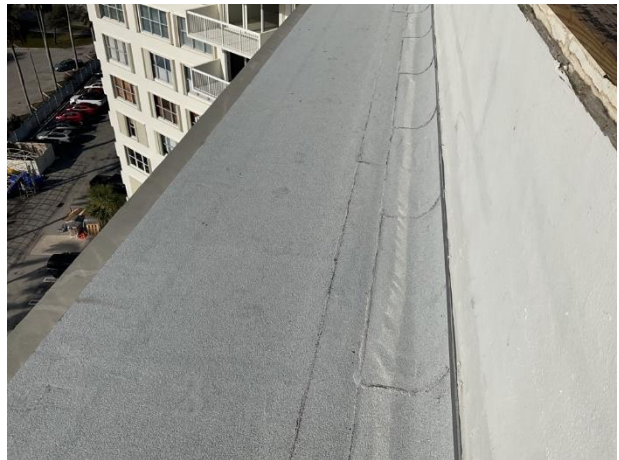
Modified bitumen roof overview
