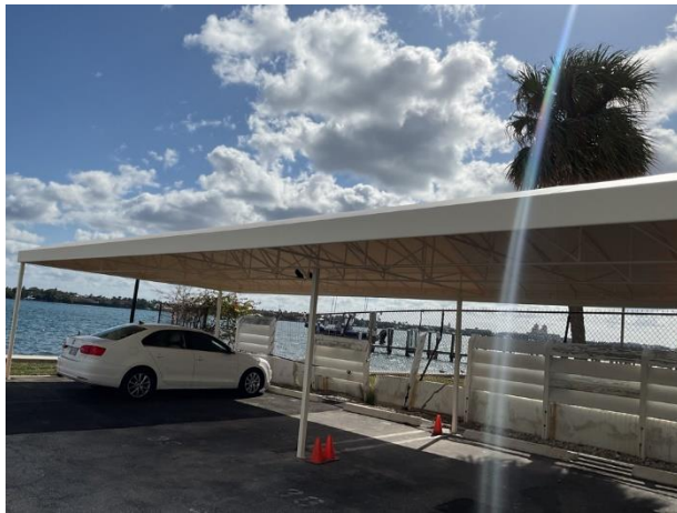
Completed section of awning
