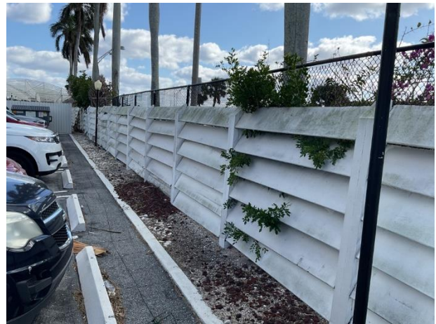
Wood fence with finish deterioration
