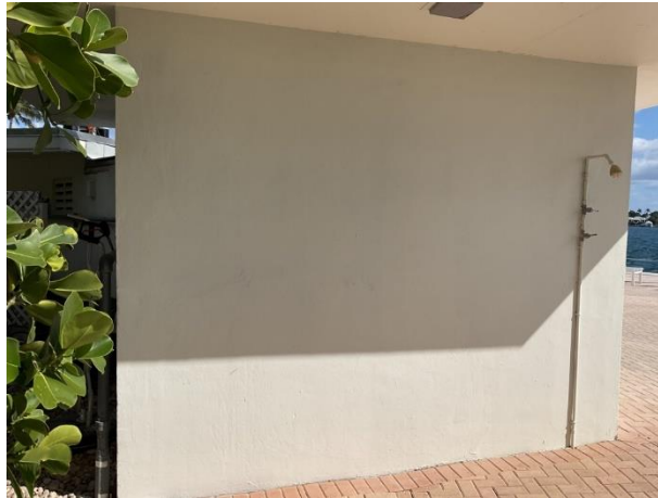
Stucco wall finishes at the pool house
