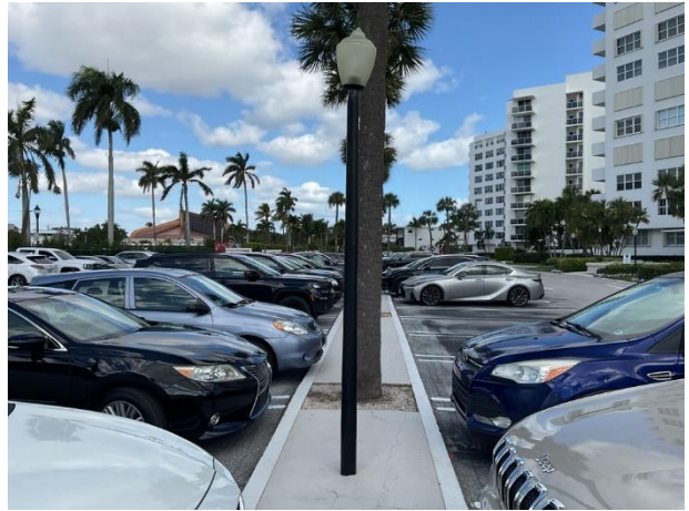
Light pole and fixture
