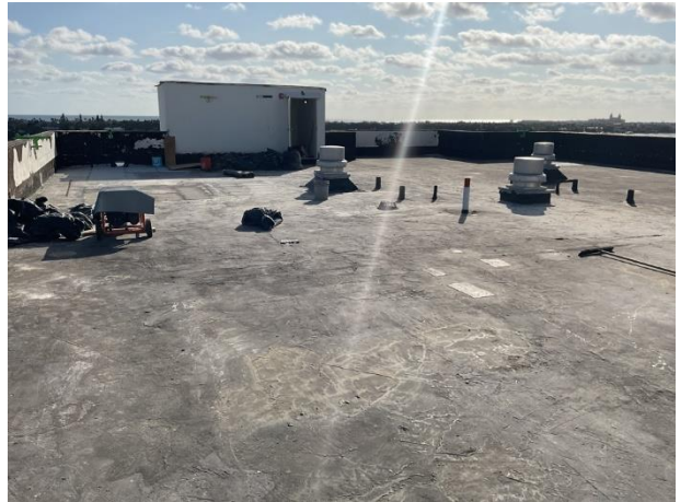
Coal tar roof overview
